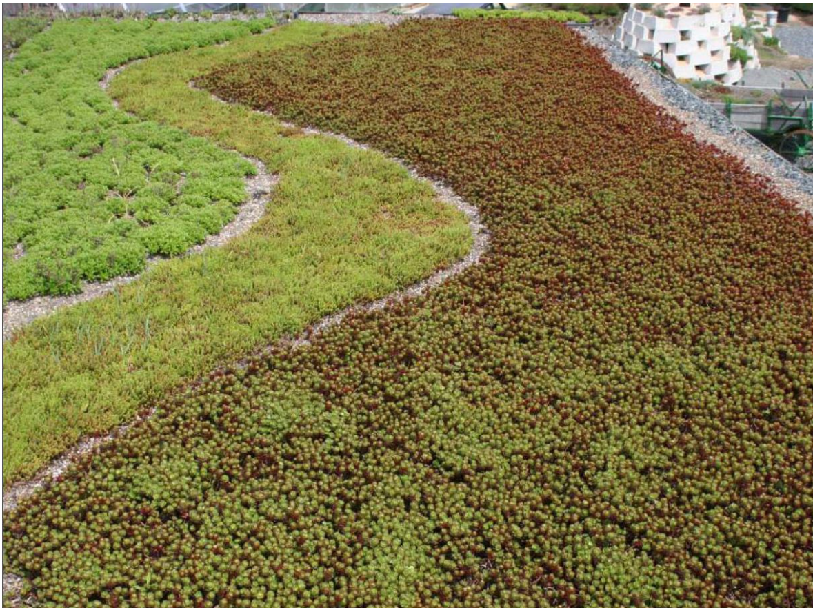
FIGURE 53: EXAMPLE OF A COMPLETED EXTENSIVE GREEN ROOF SYSTEM (PASCHAL, 2006)
